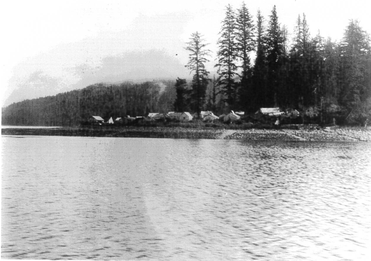
Figure 2. This image was taken from the south end of Shaanda across Shaan Seet toward the Cannery Point village. The structures at the point on the left appear to have been replaced with more permanent structures. With possible exception of most recent apparent structures that appear to be of a more permanent basis using American architectural principles that are partially hidden by the woods on the right of the picture, the other structures appear to be of more traditional camp-style construction based on the presence of the smoke hole in the roof of the structure.
