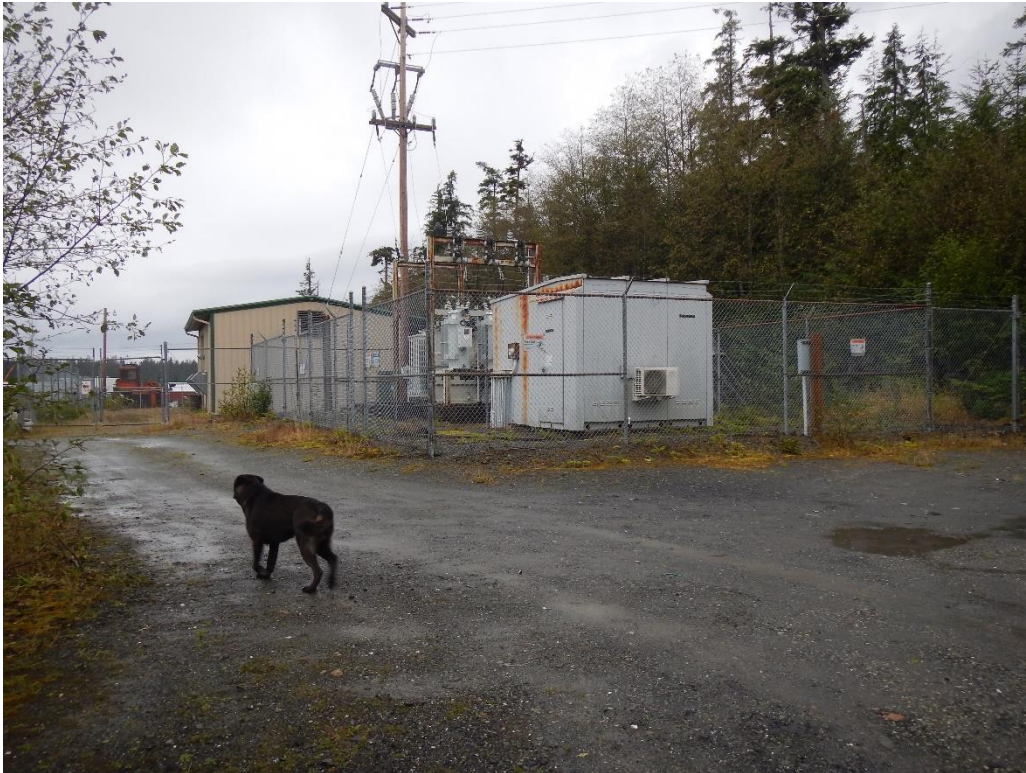
Looking west over Lot 6, JT Brown Park, AP&T Lease (100920-77)
