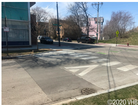
Figure 2. Photo. Raised crosswalk in Chicago with additional drainage grates added upstream of crossing.
