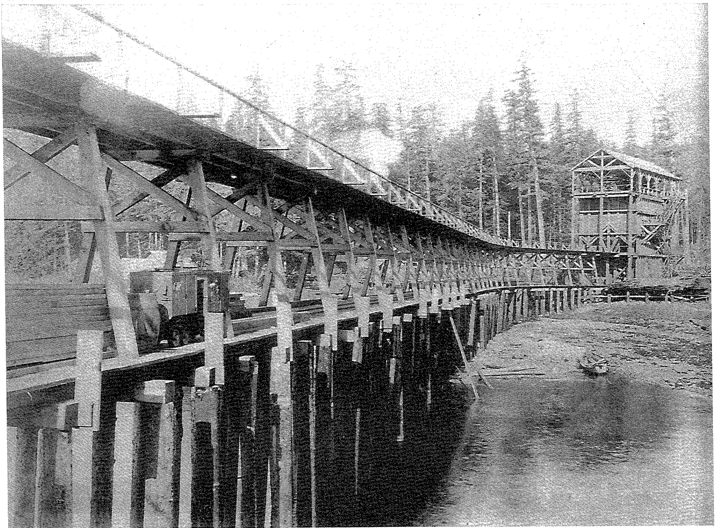
Historical infrastructure at Niblack on Prince of Wales Island.
