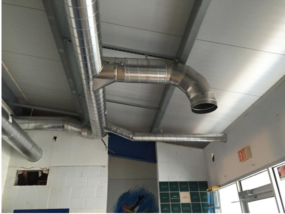
New Ductwork in Lobby 7-15-16
