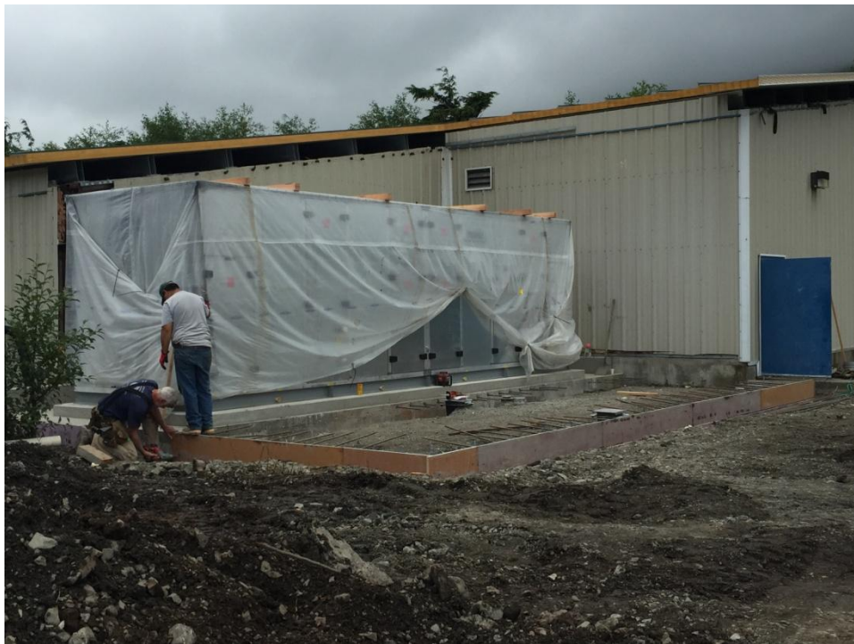
New AHU-1 Installed on Pad 7-15-16
