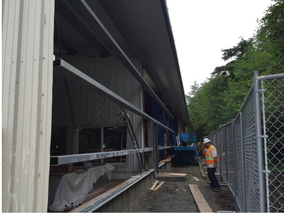
East Wall Demolition and Reconstruction 7-15-16
