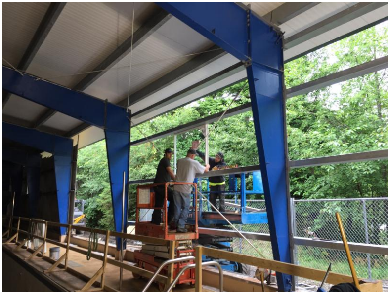
Setting a new window in the East Wall
