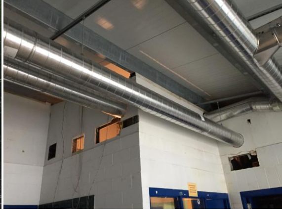
New Ducting in the Lobby
