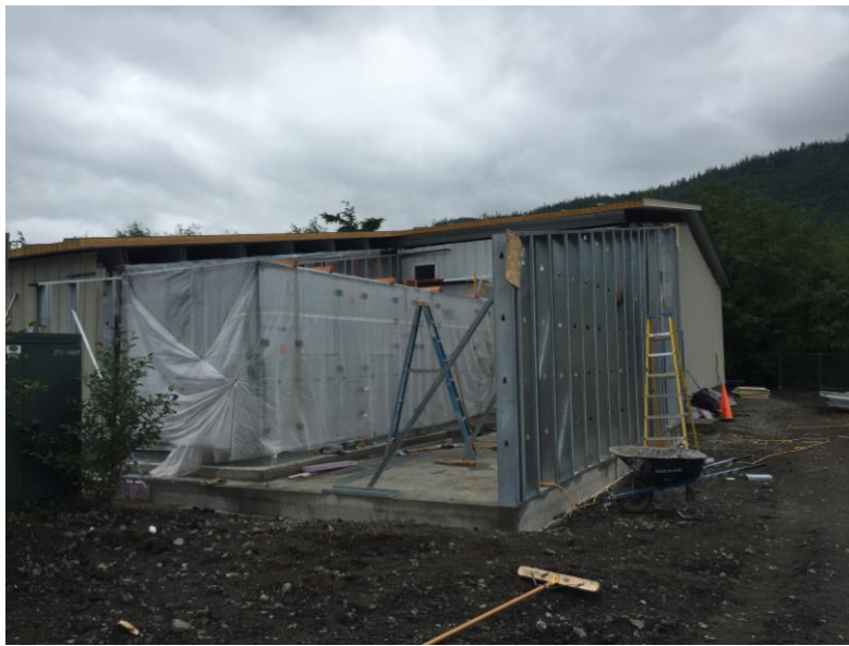
New AHU I and Mechanical Room Framing
