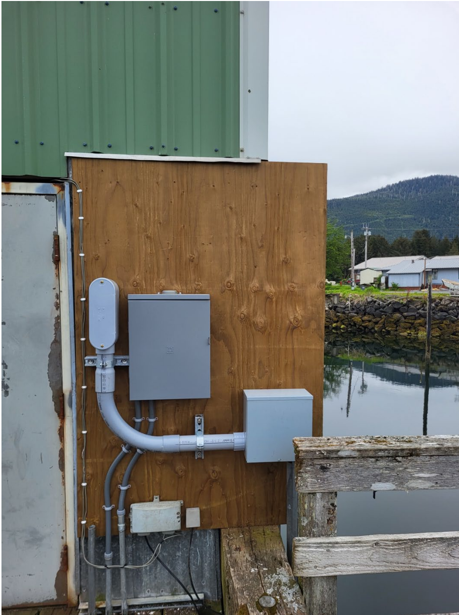
New plywood against building, and new rain tight service panel.
