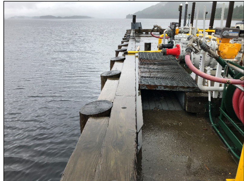
Timber bullrail/curb and fender piles at dock face.
