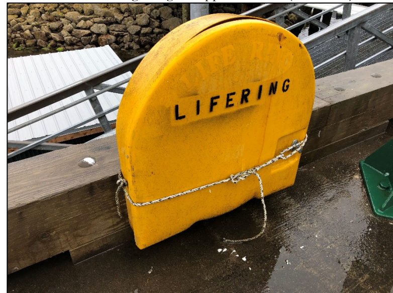
Life ring cabinet w/ broken door hinge assembly.
