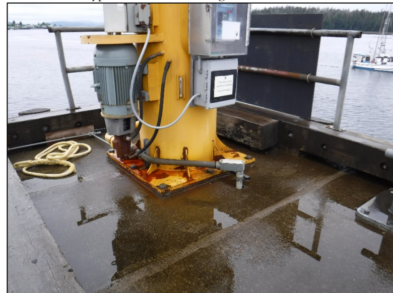
Crane base on concrete deck.
