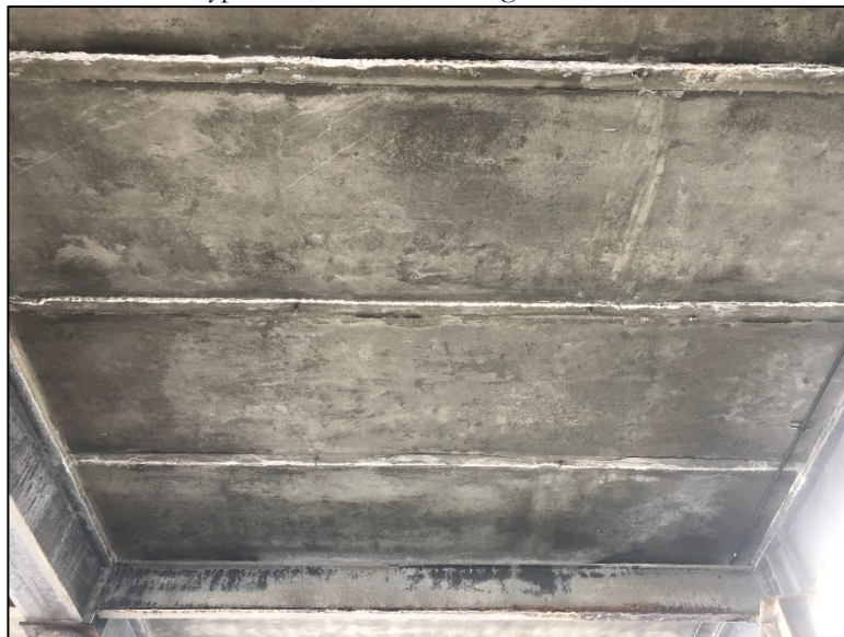
Typical concrete deck panels under dock.
