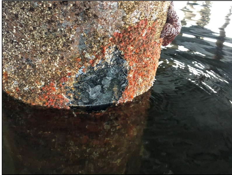
Typical dock support pile surface condition in tidal zone.
