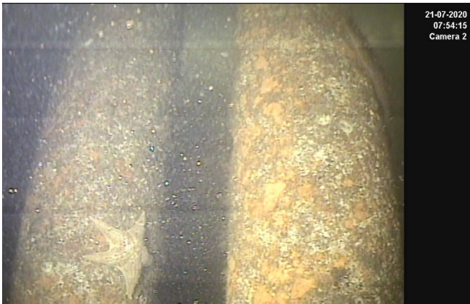
INDUSTRIAL DOCK: Steel pile
