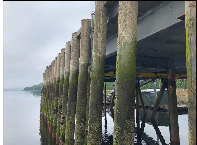
Overview of timber fender piles along dock face.
