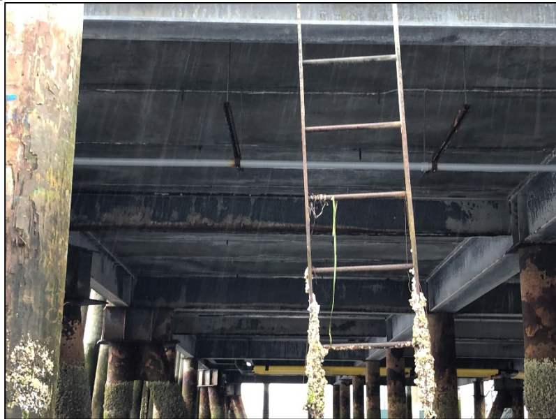
Typical steel dock framing under dock.
