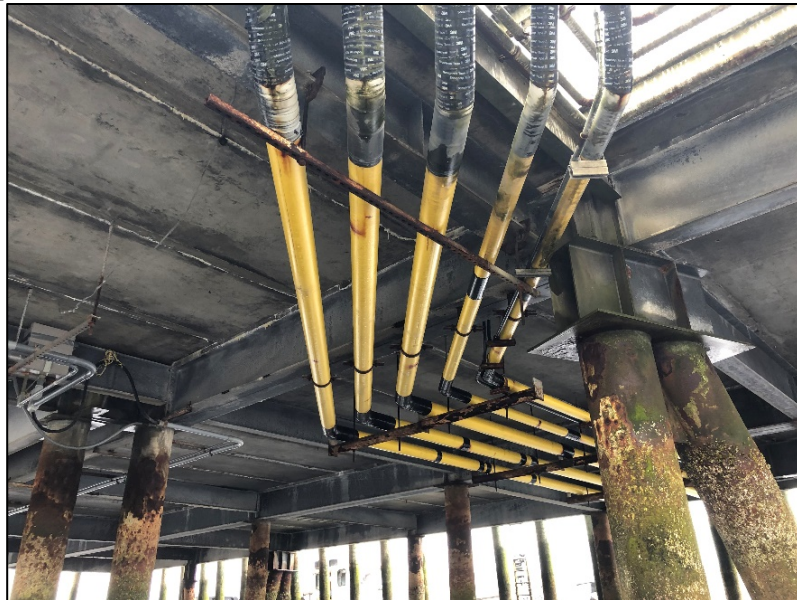
Fuel line routing under dock at approach/main dock junction.
