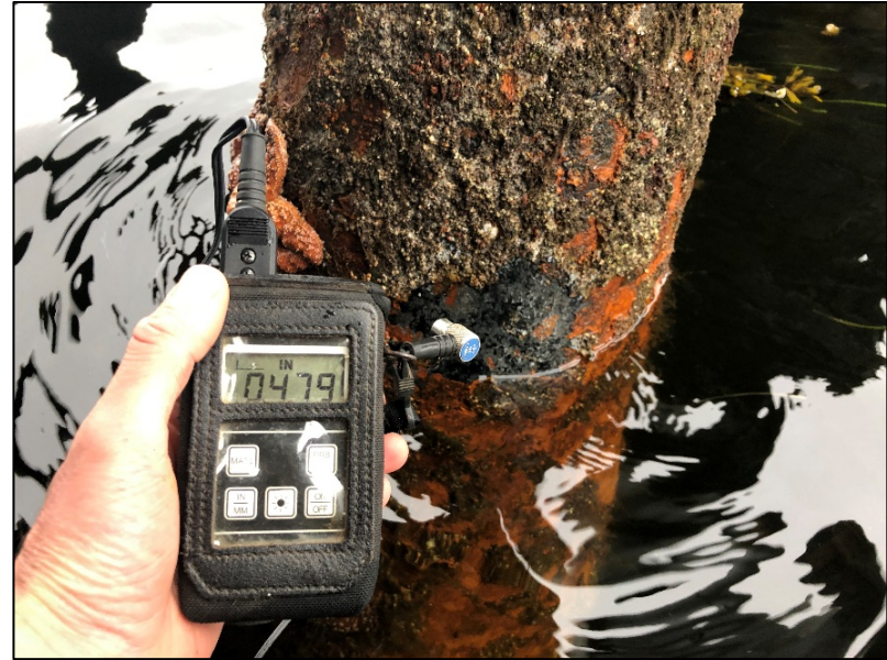
Steel dock pile thickness measurement.
