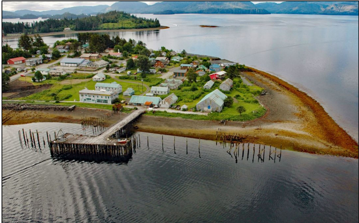
Figure 2: Current Structures Within Project Area
