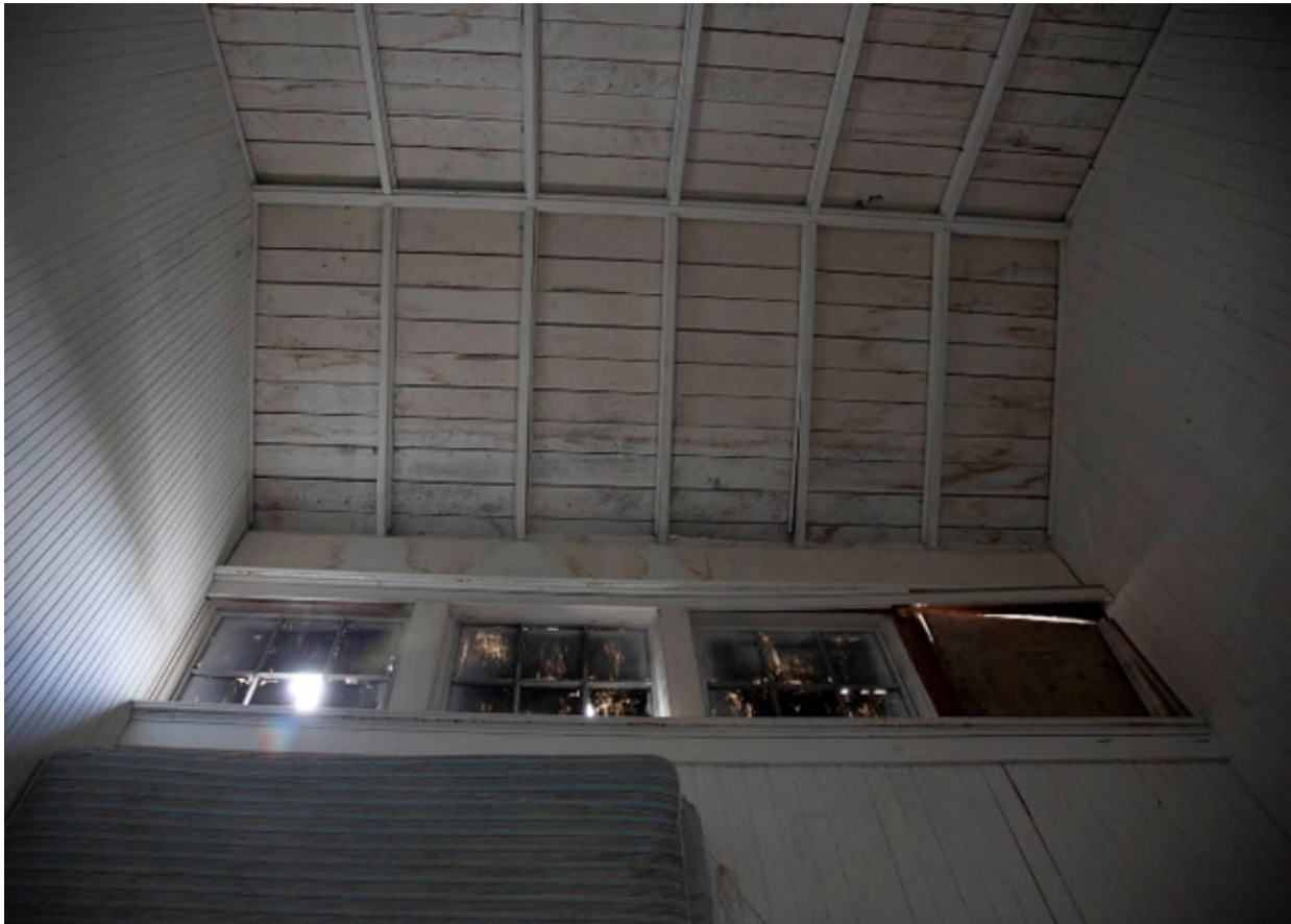
Figure 13. Administrative Building Roof Projection. View from Interior.
