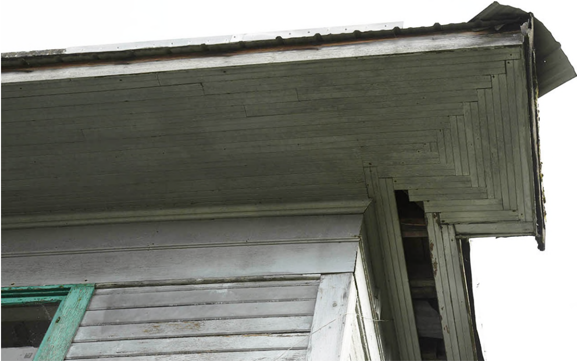
Figure 14. Administrative Building, Cornice Detail.
