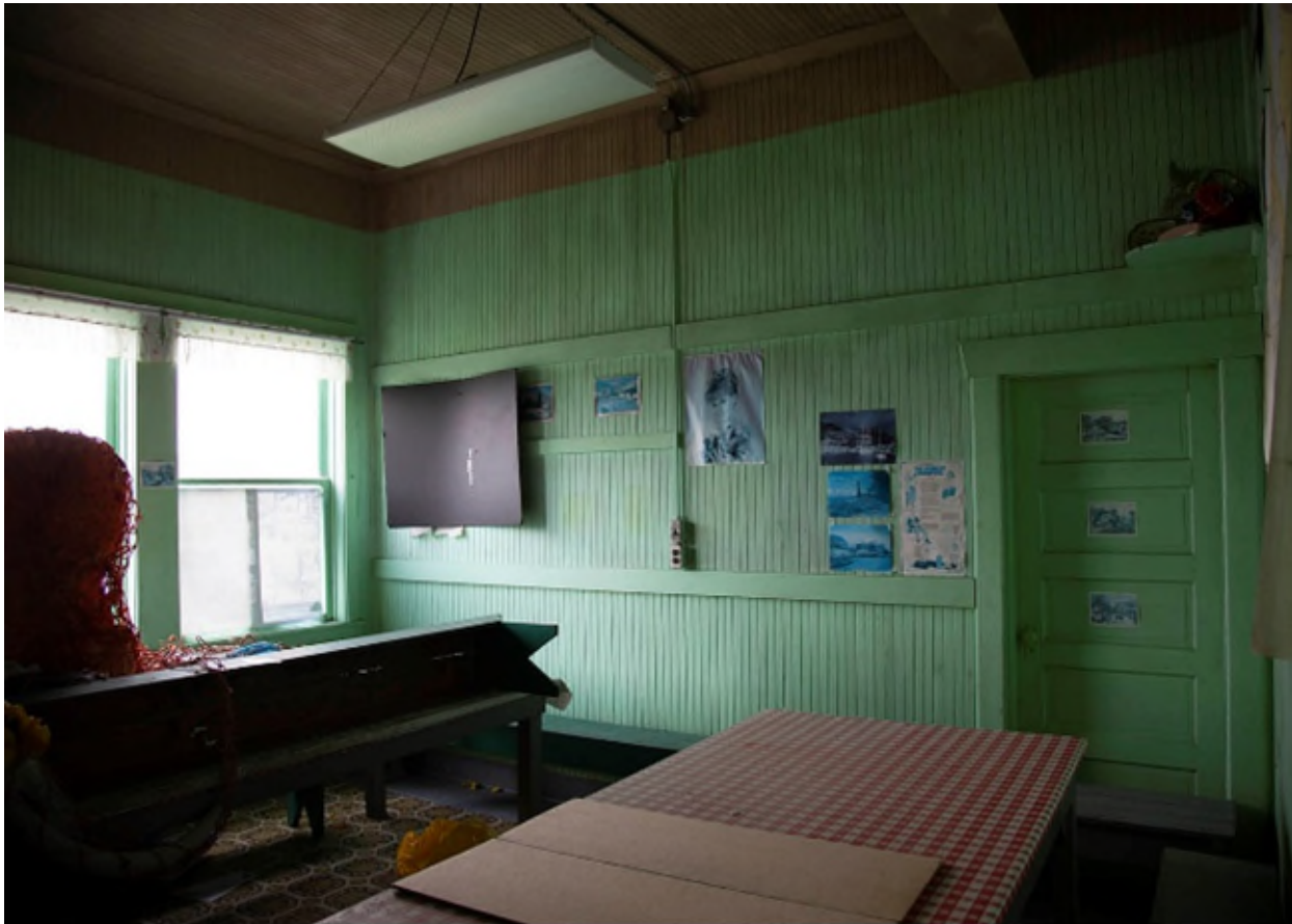
Figure 17. Administrative Building Dining Room, First Story. View Looking NE.
