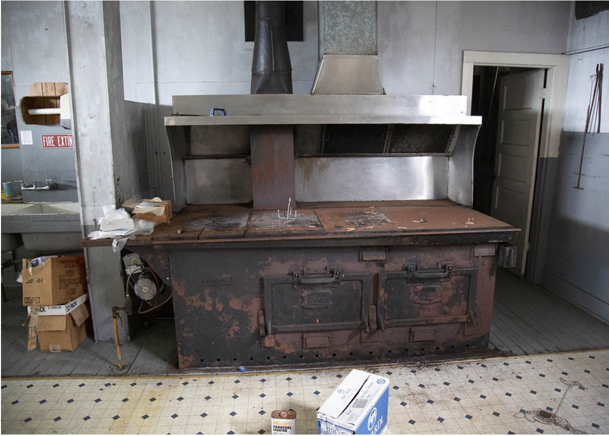
Figure 18. Administrative Building Commercial Range and Kitchen, First Story.
