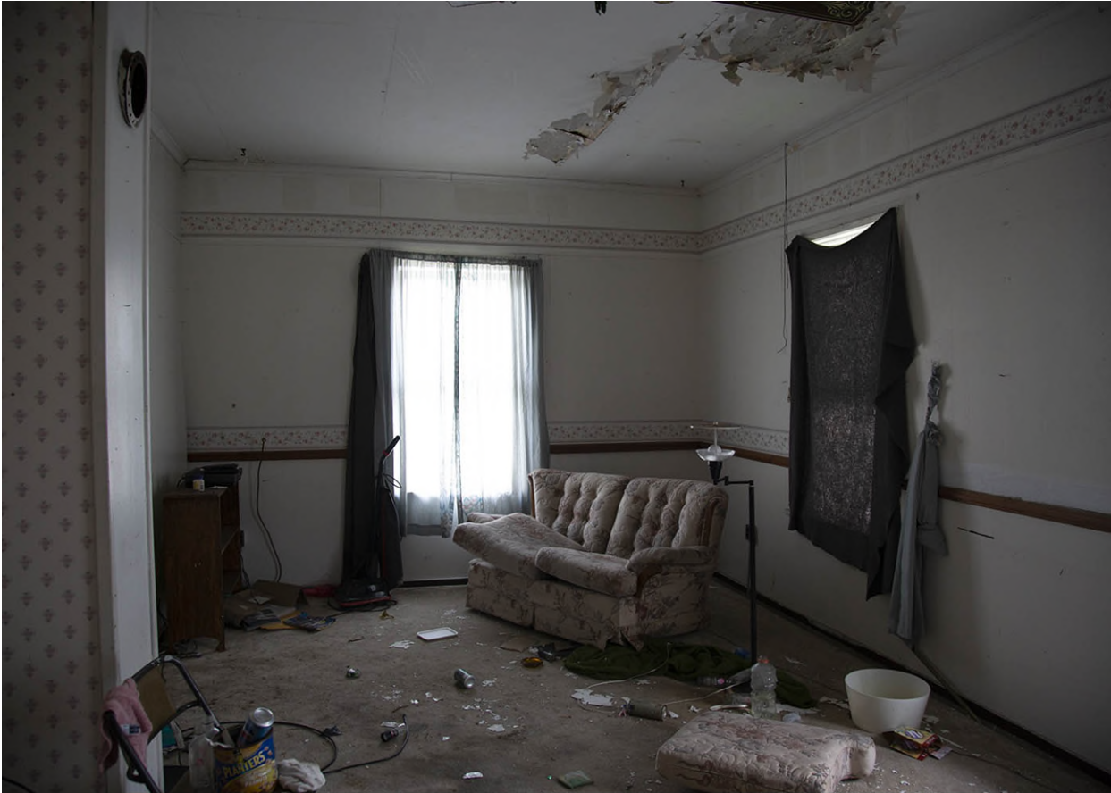
Figure 26. Administrative Building, Second Story Room.
