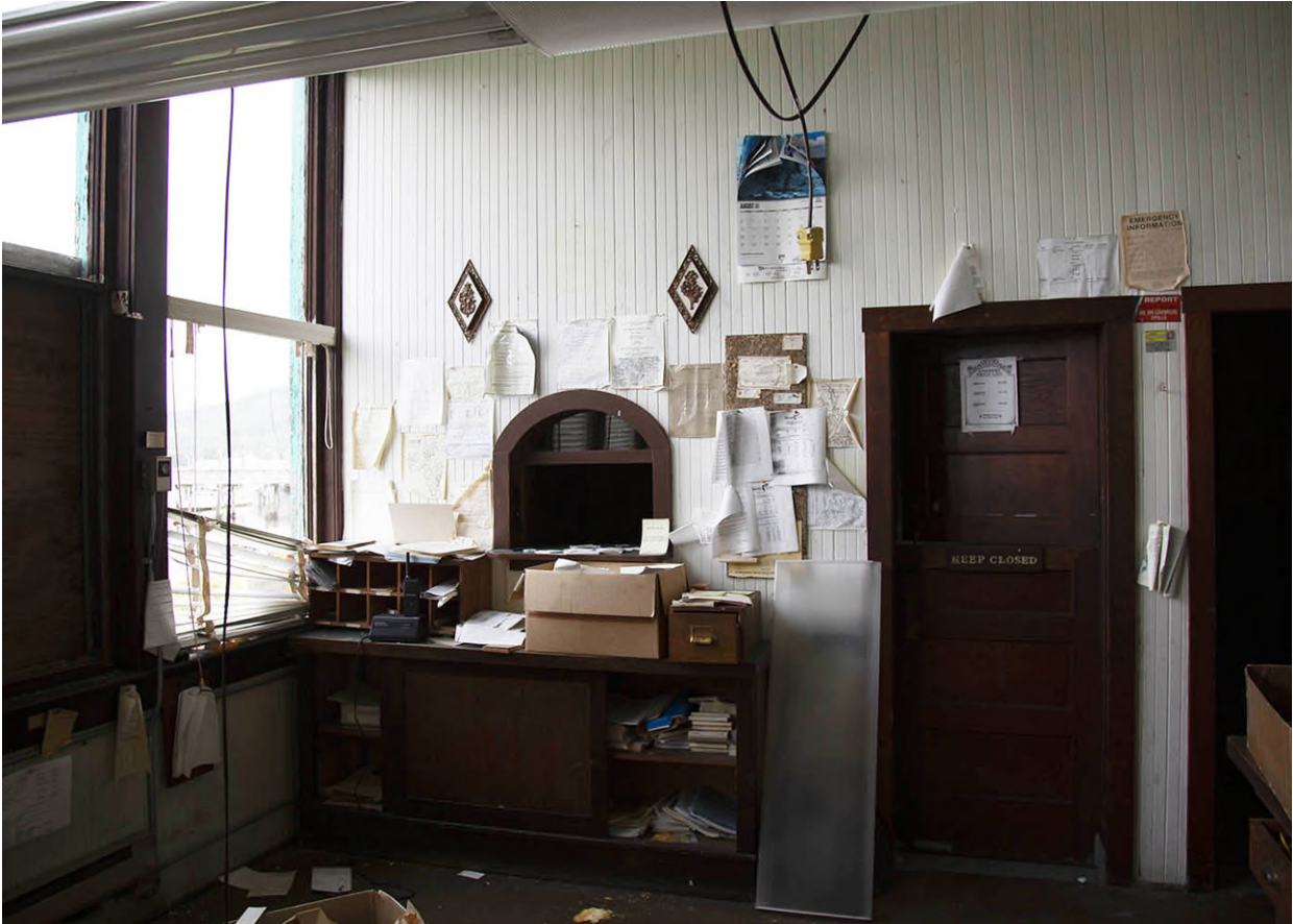
Figure 23. Administrative Building Fish Ticket Window, First Story.
