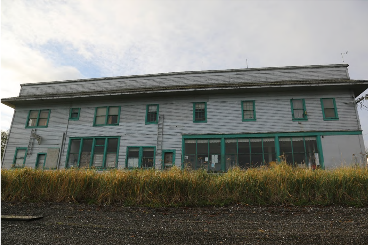
Figure 2. Primary (North) Facade of Administrative Building. View Looking S.
