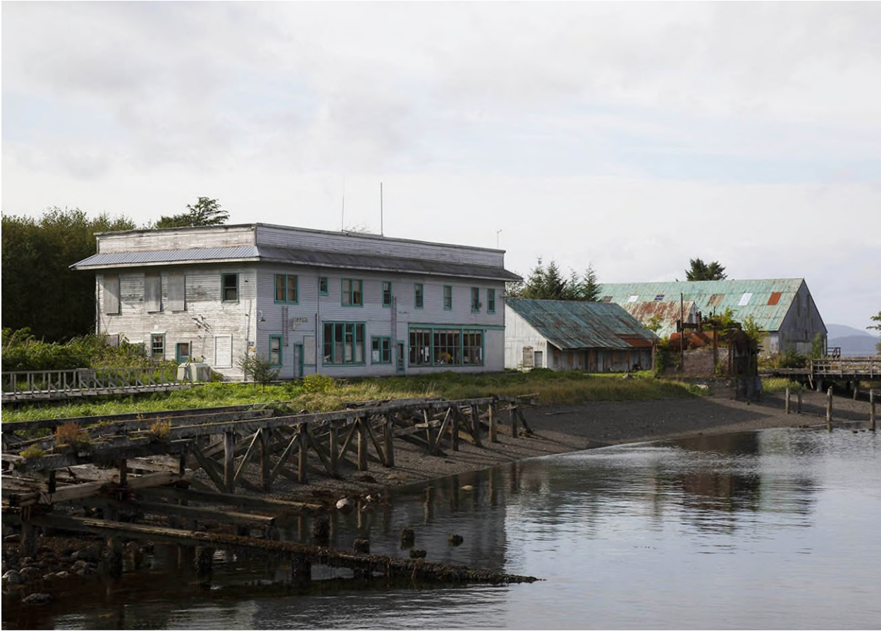
Figure 6. Administrative Building, Maintenance Building and Web Loft. View Looking S.W.
