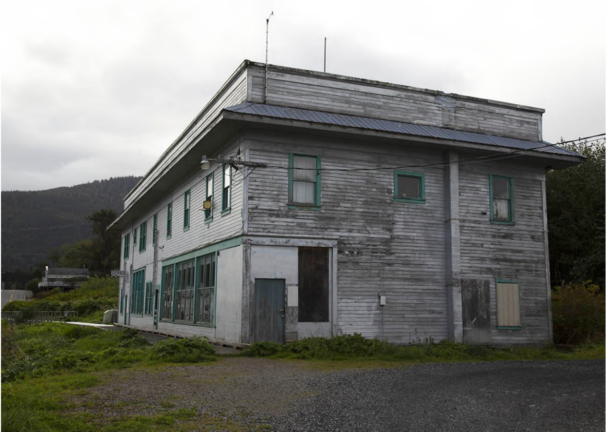
Figure 3. West and North Facades of Administrative Building. View Looking E.
