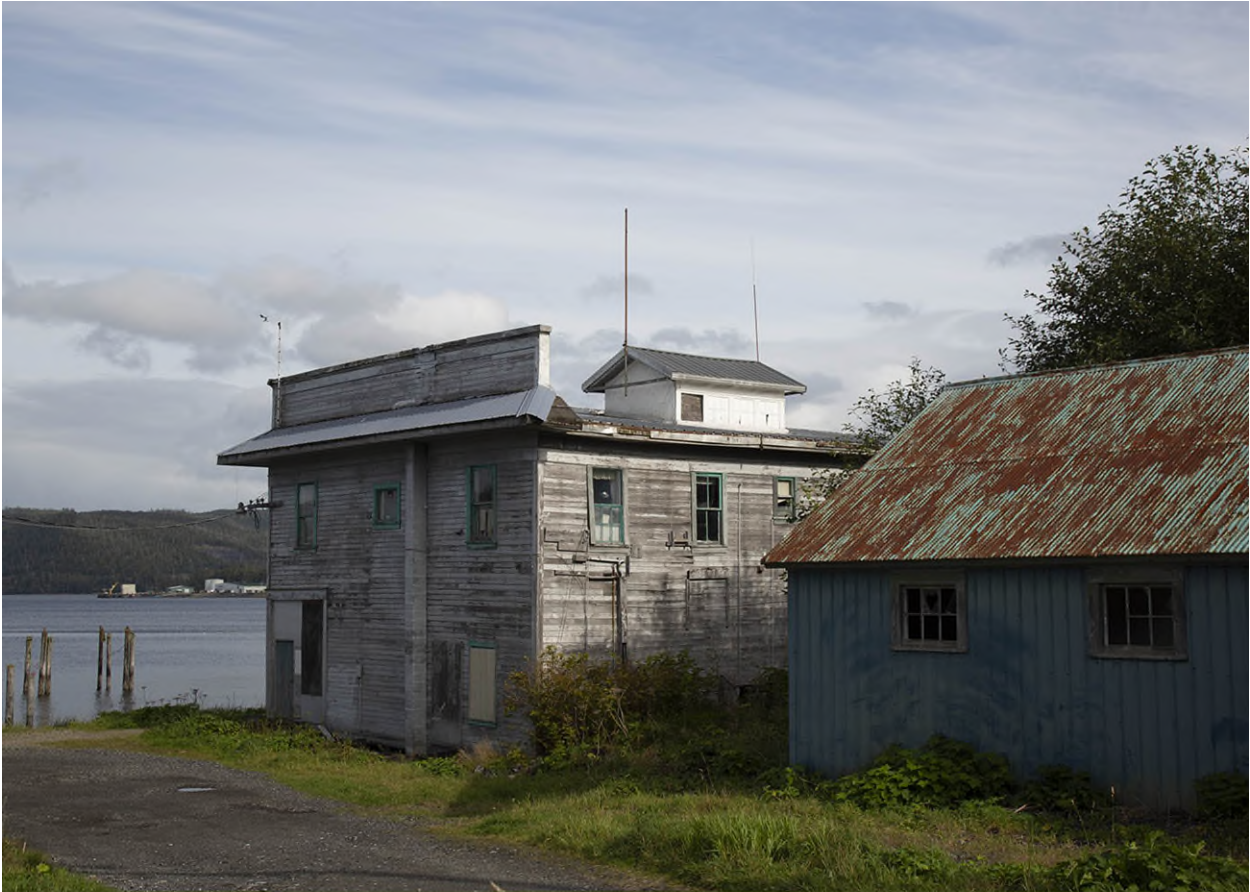
Figure 9. Administrative Building Roof Projection with Clerestory Windows. View N.
