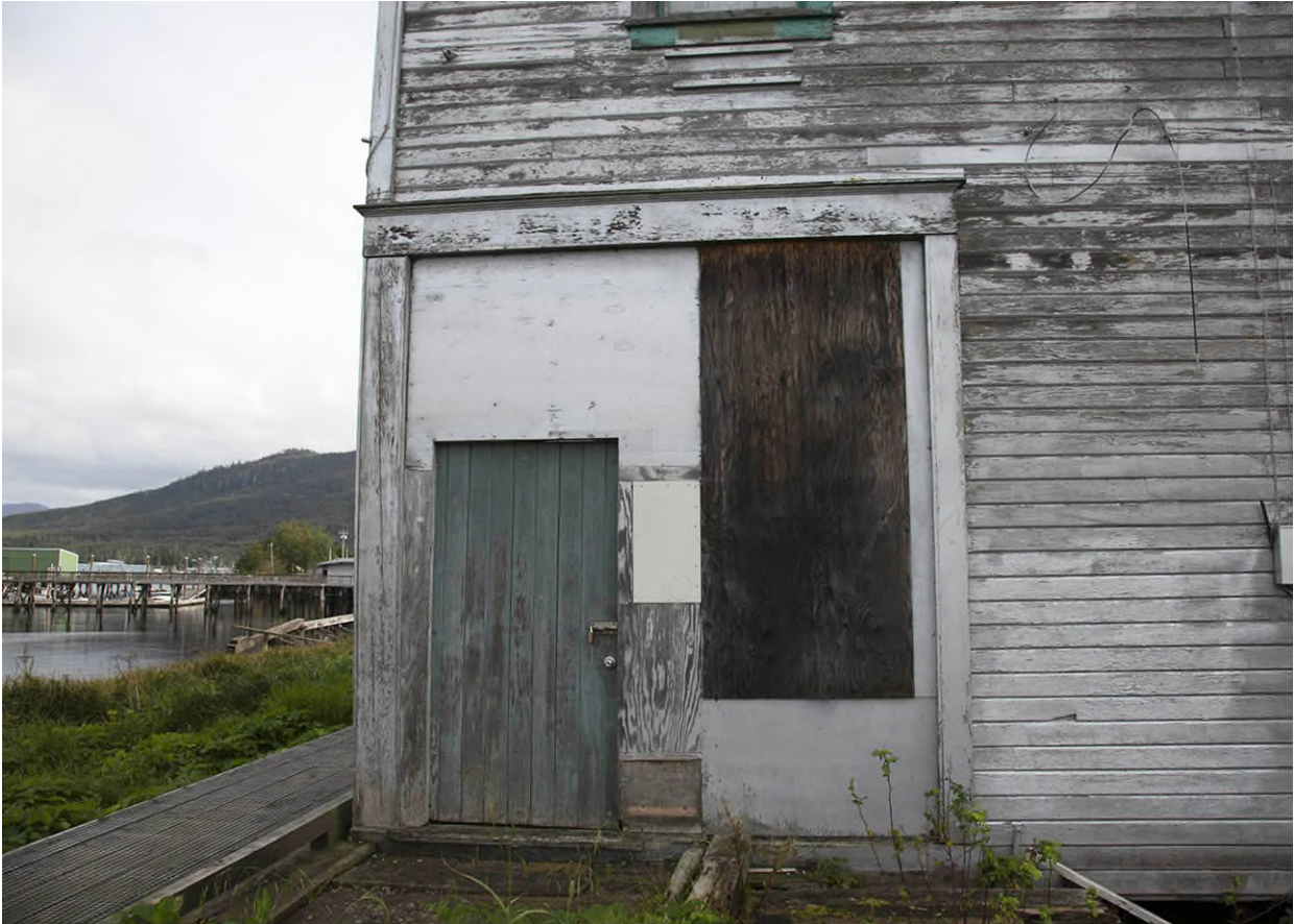
Figure 8. Enclosed Primary Entry. View Looking E.
