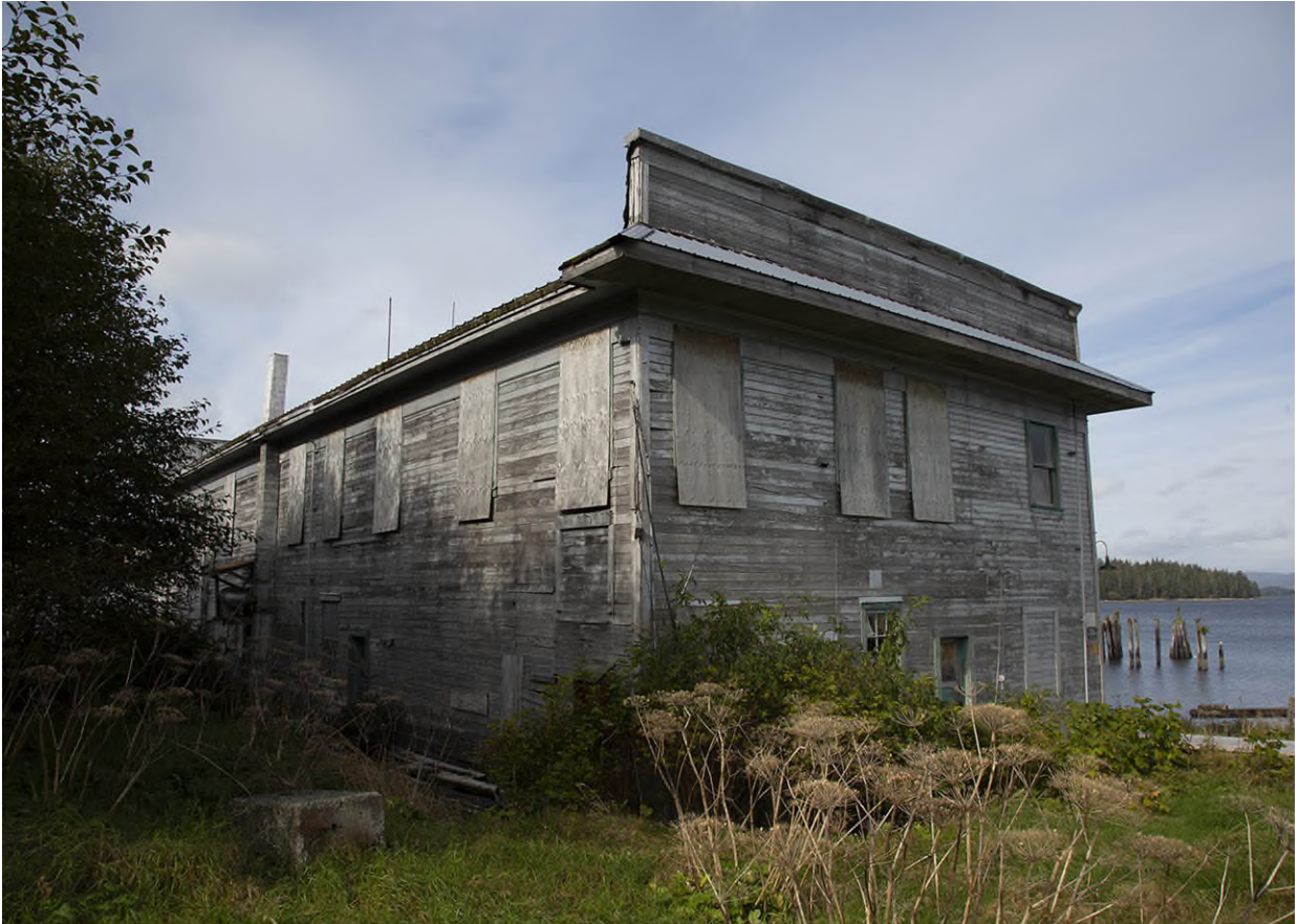
Figure 5. East and South Facades of Administrative Building. View Looking N.W.
