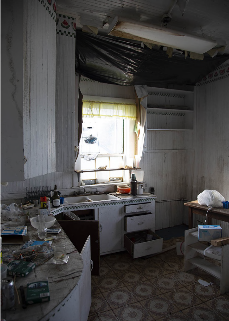
Figure 28. Administrative Building, Second Story Kitchen.
