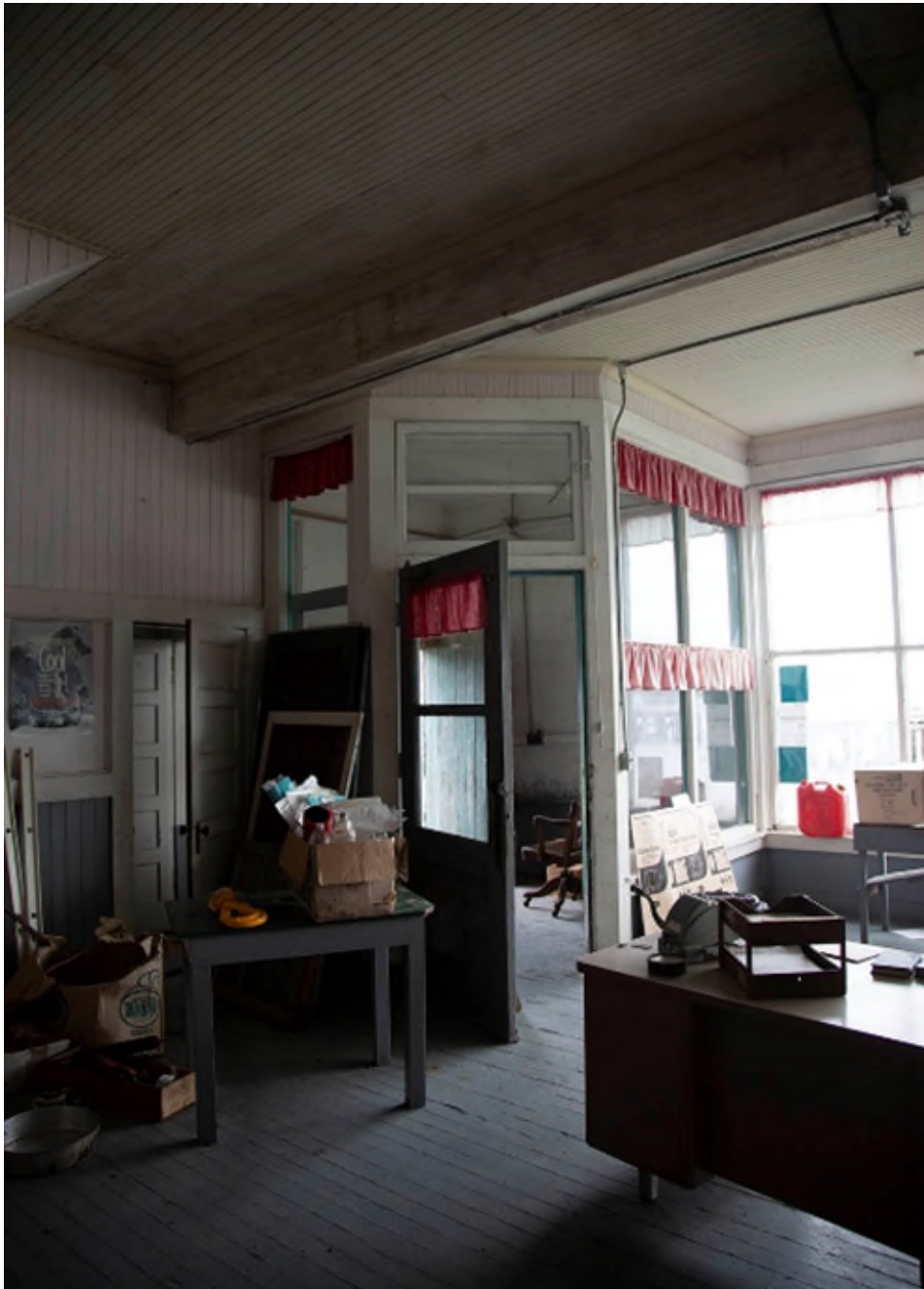
Figure 12. Primary Entry From Interior. View N.W.
