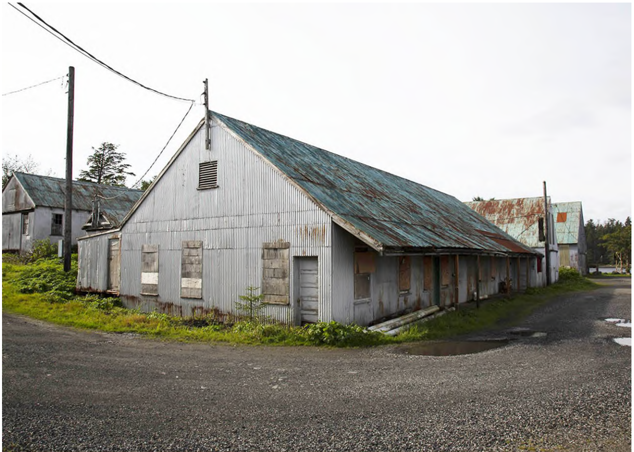
Figure 3. Maintenance Building, North and East Facades. View Looking W.
