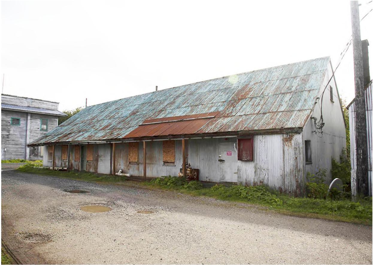
Figure 1. Maintenance Building, North (Primary) and West Facades. View looking S.E.
