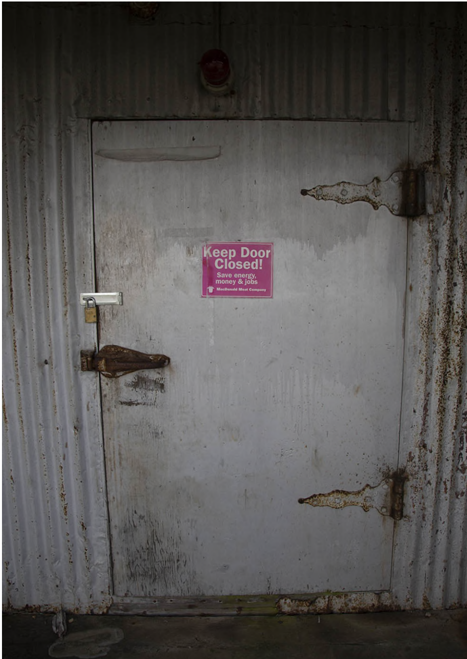
Figure 7. Maintenance Building, Cold Storage Door. View Looking S.
