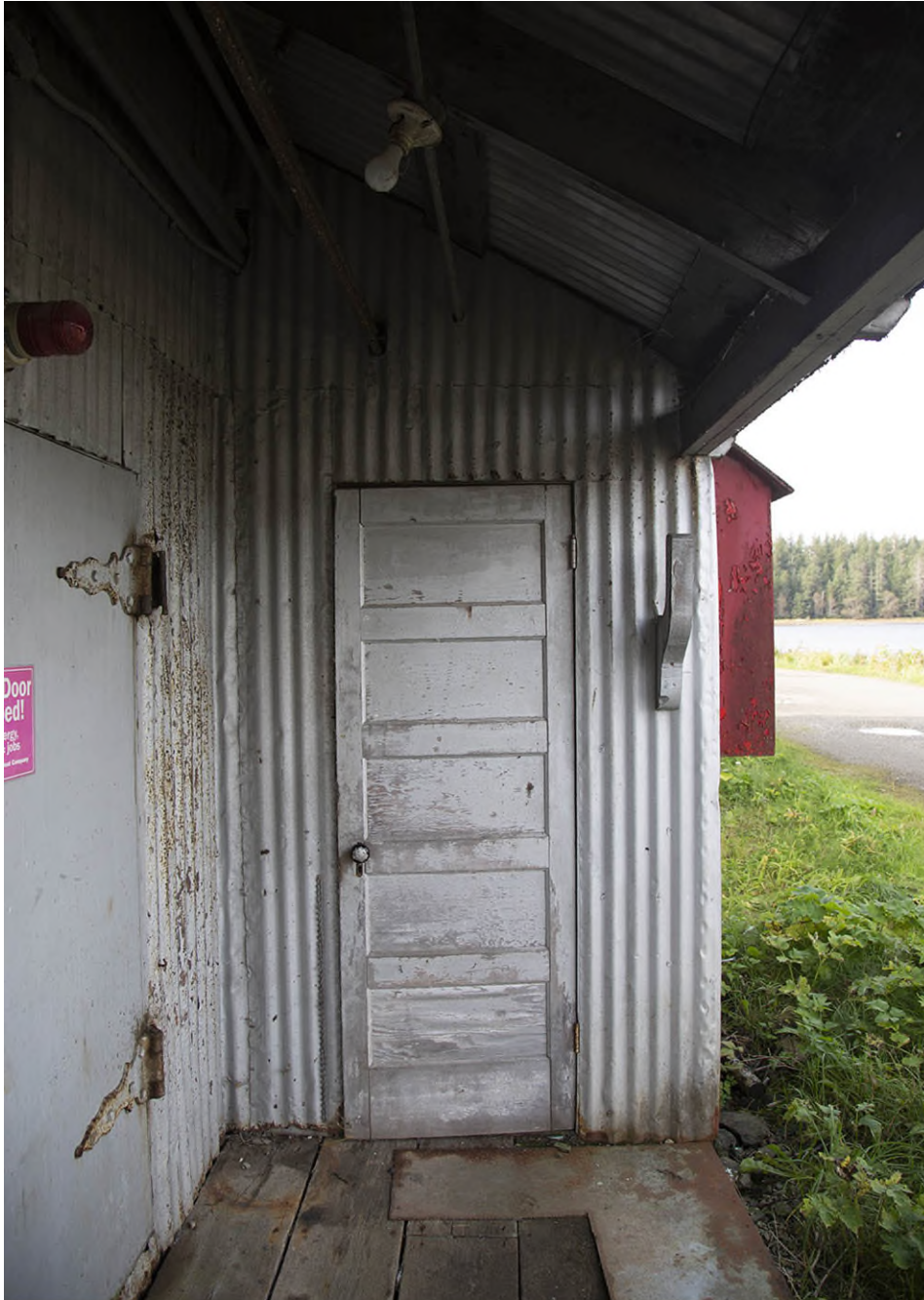
Figure 6. Maintenance Building, Representative Paneled Wood Door. View Looking W.
