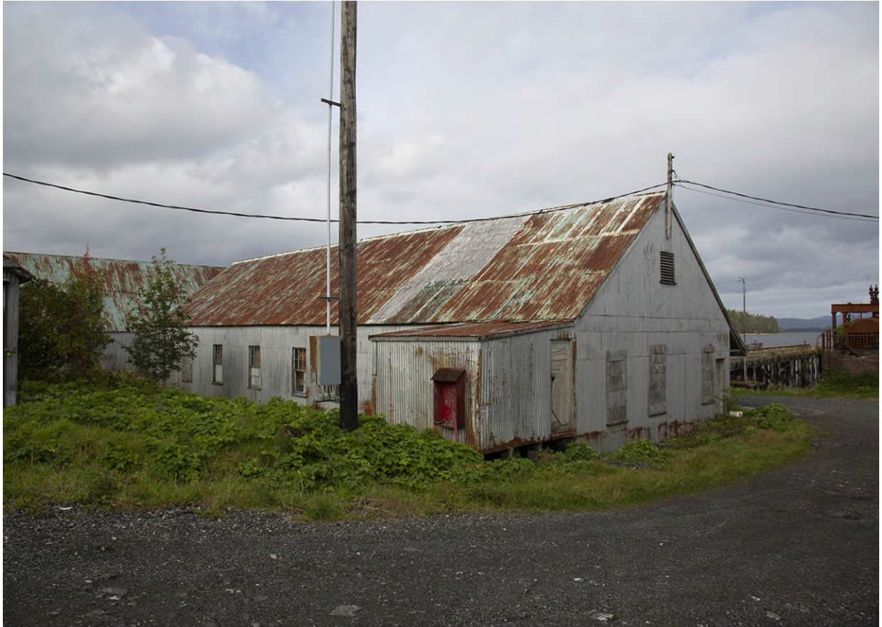
Figure 5. Maintenance Building, South and East Facades. View Looking N.
