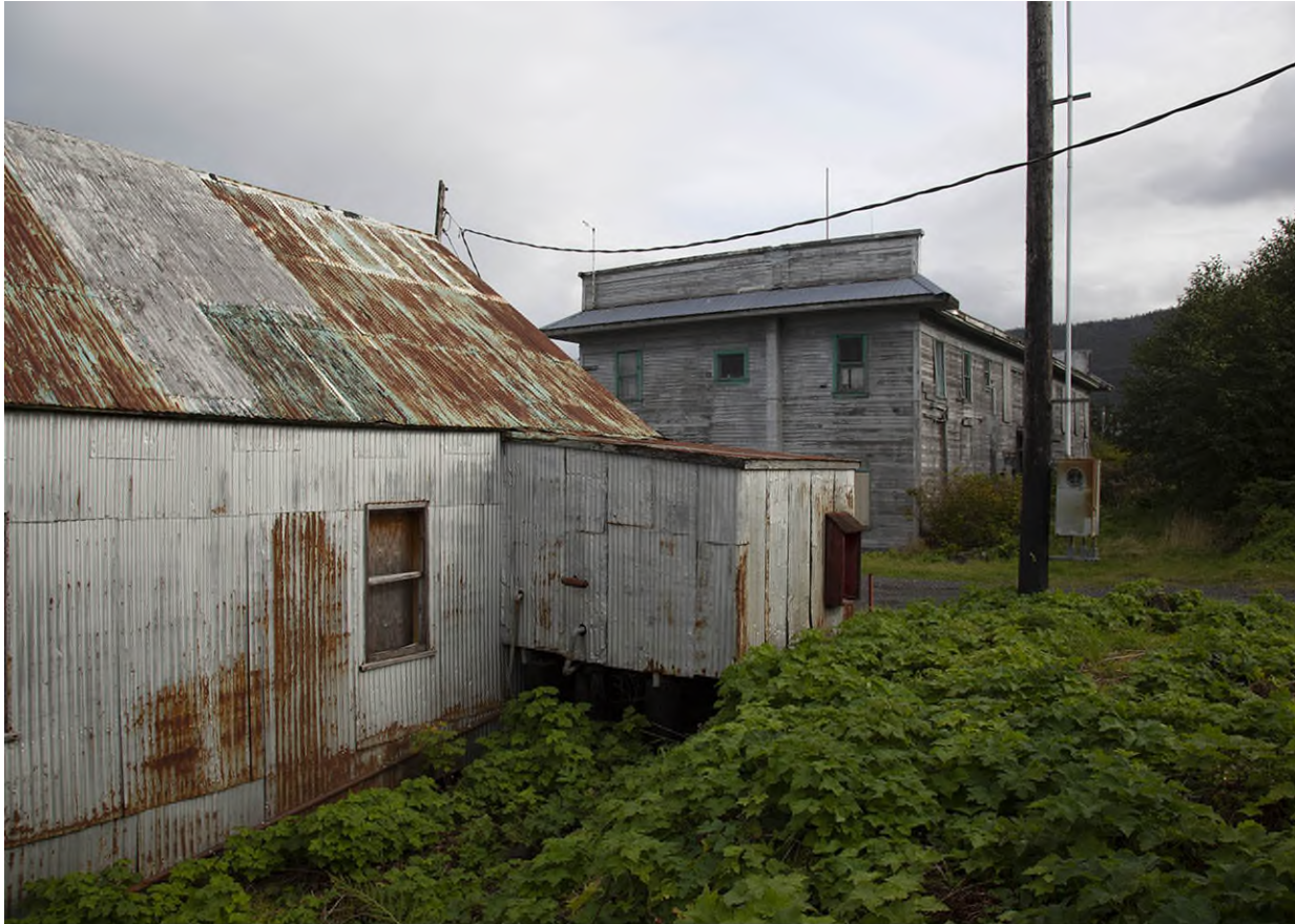
Figure 11. Maintenance Building, Southeast Corner Projection. View Looking E.
