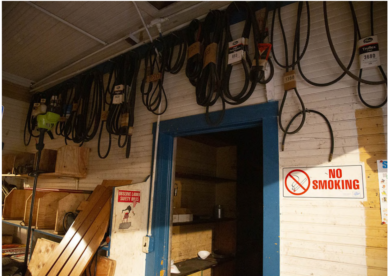
Figure 15. Maintenance Building, Interior. View Looking E.
