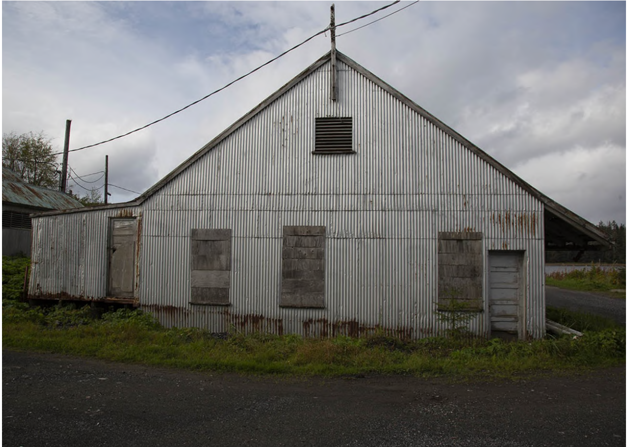
Figure 4. Maintenance Building, East Facade. View Looking W.
