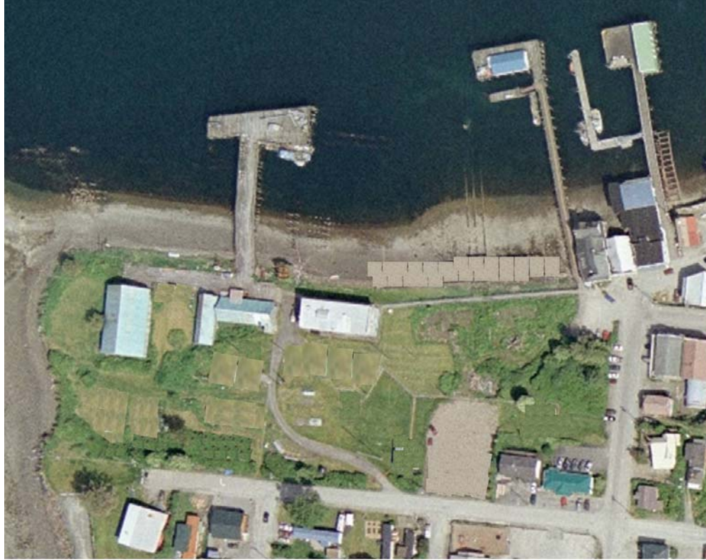
Figure 2, Ward Cove Cannery Site with Designated Buildings Removed
