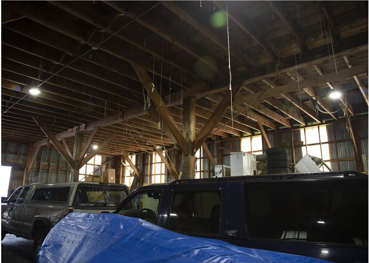
Figure 8. Web Loft, Interior of First Floor, East Wall. View Looking NE.
