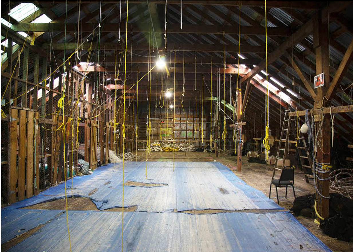
Figure 9. Web Loft, Interior Half Story (Loft). View Looking S.
