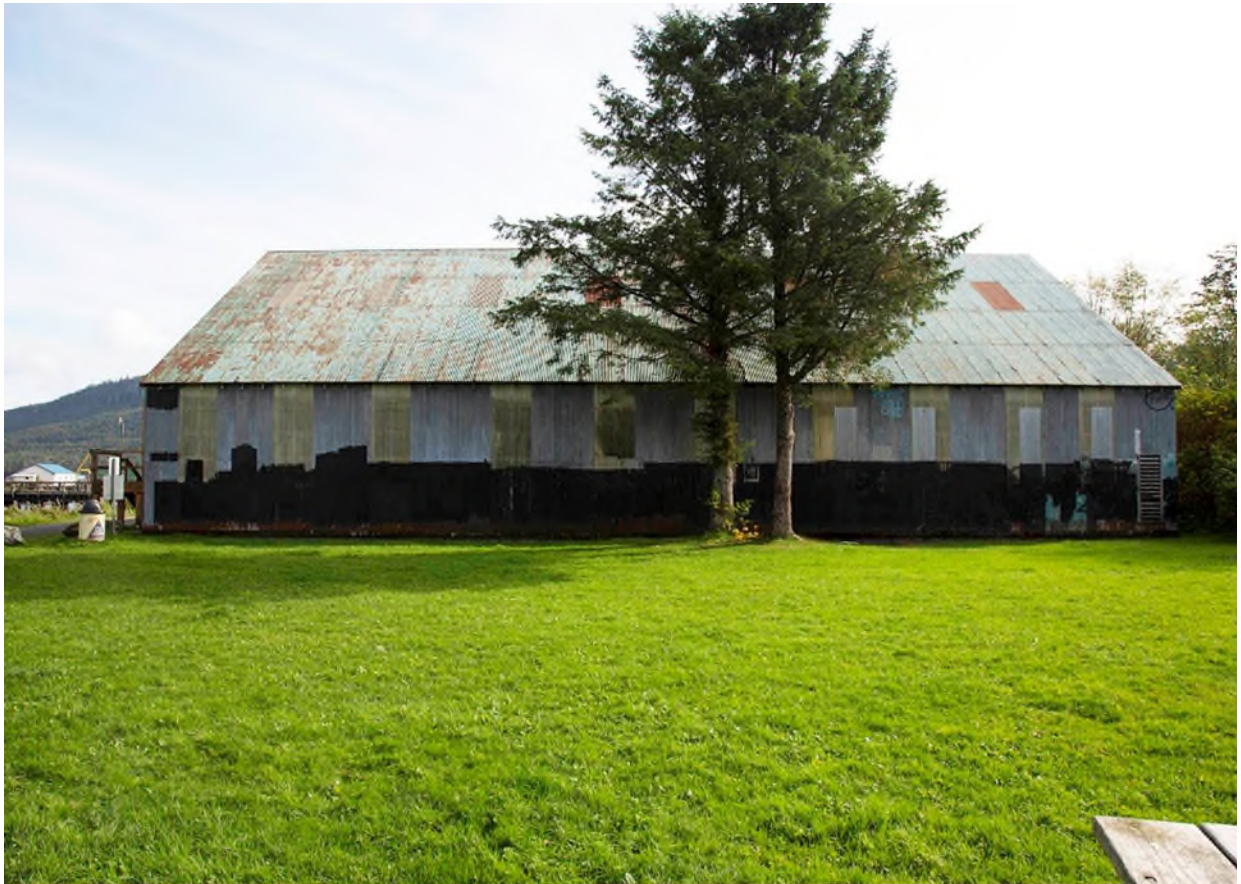
Figure 5. Web Loft, West Facade. View Looking E.
