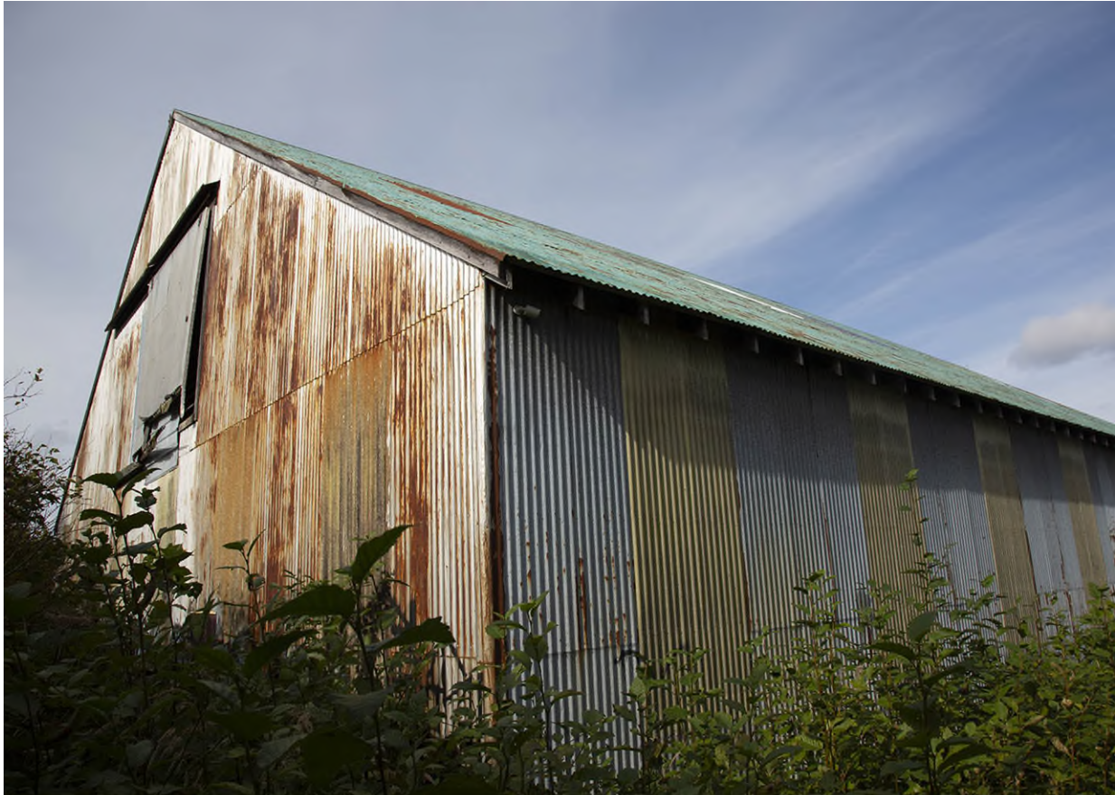
Figure 6. Web Loft, South and East Facades. View Looking N.W.
