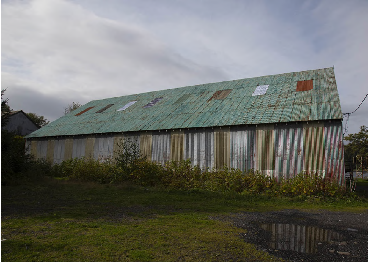
Figure 3. Web Loft, East Facade. View Looking W.
