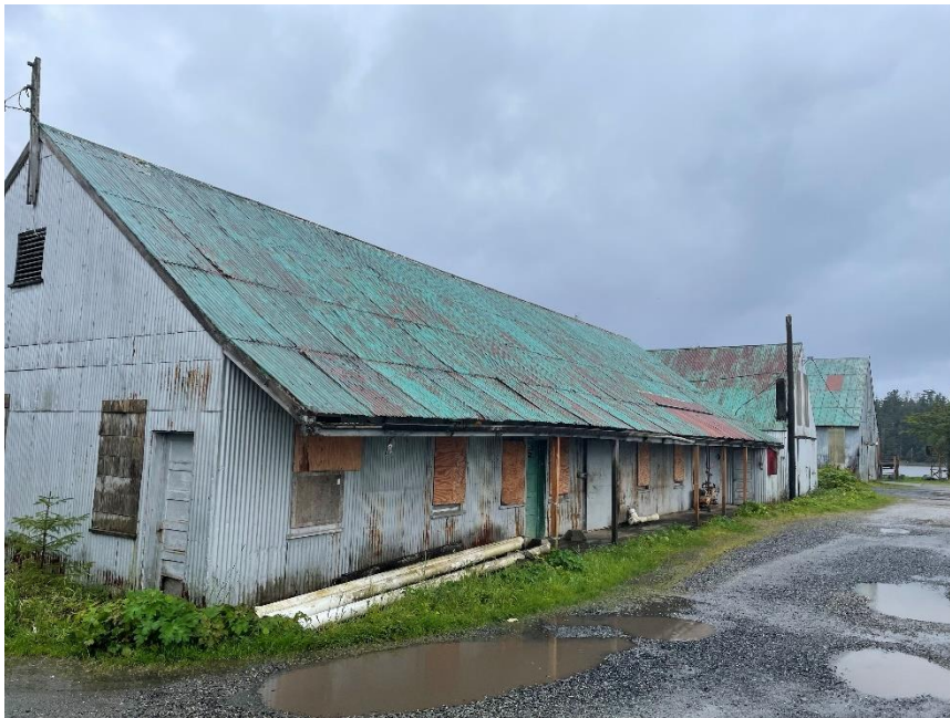
View from the North-east corner
