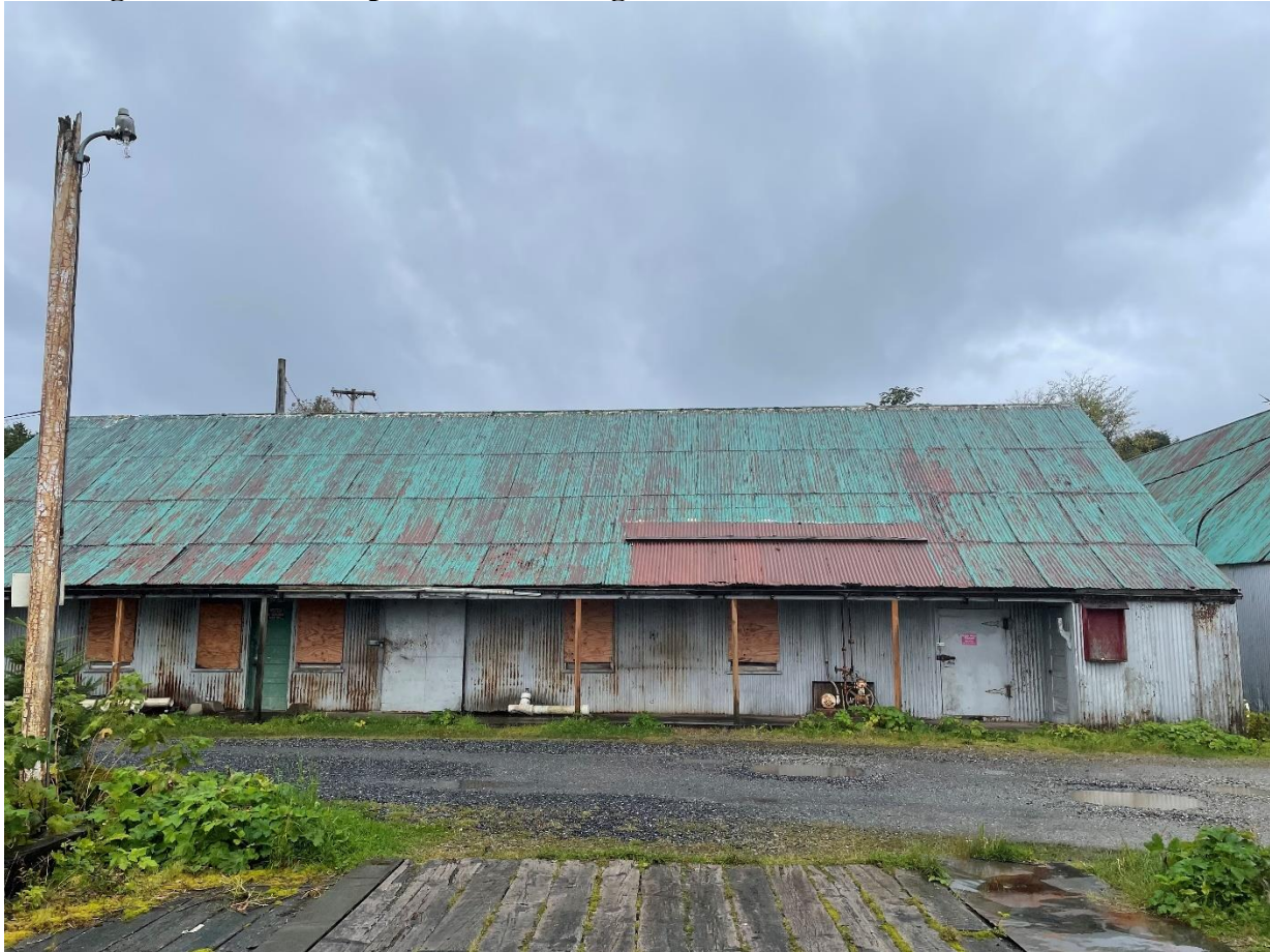
North elevation facing waterfront
