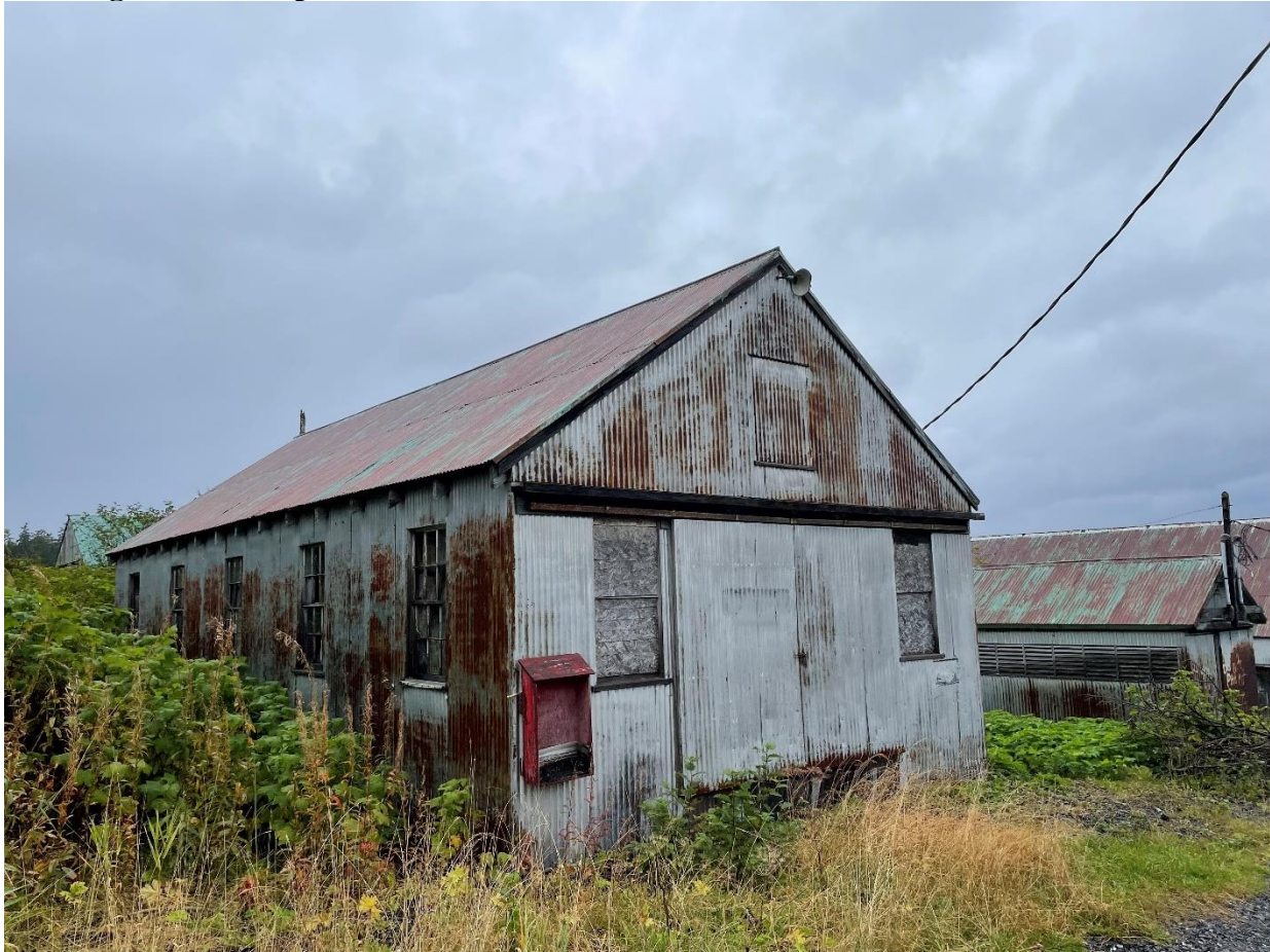
Southeast corner view
