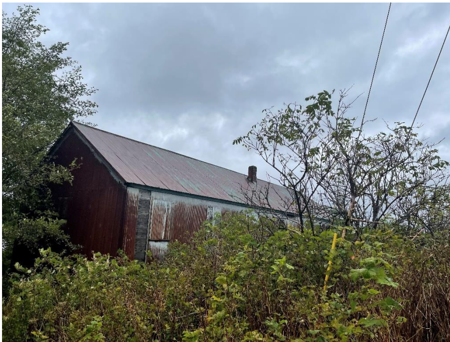
Bunkhouse, southeast corner
