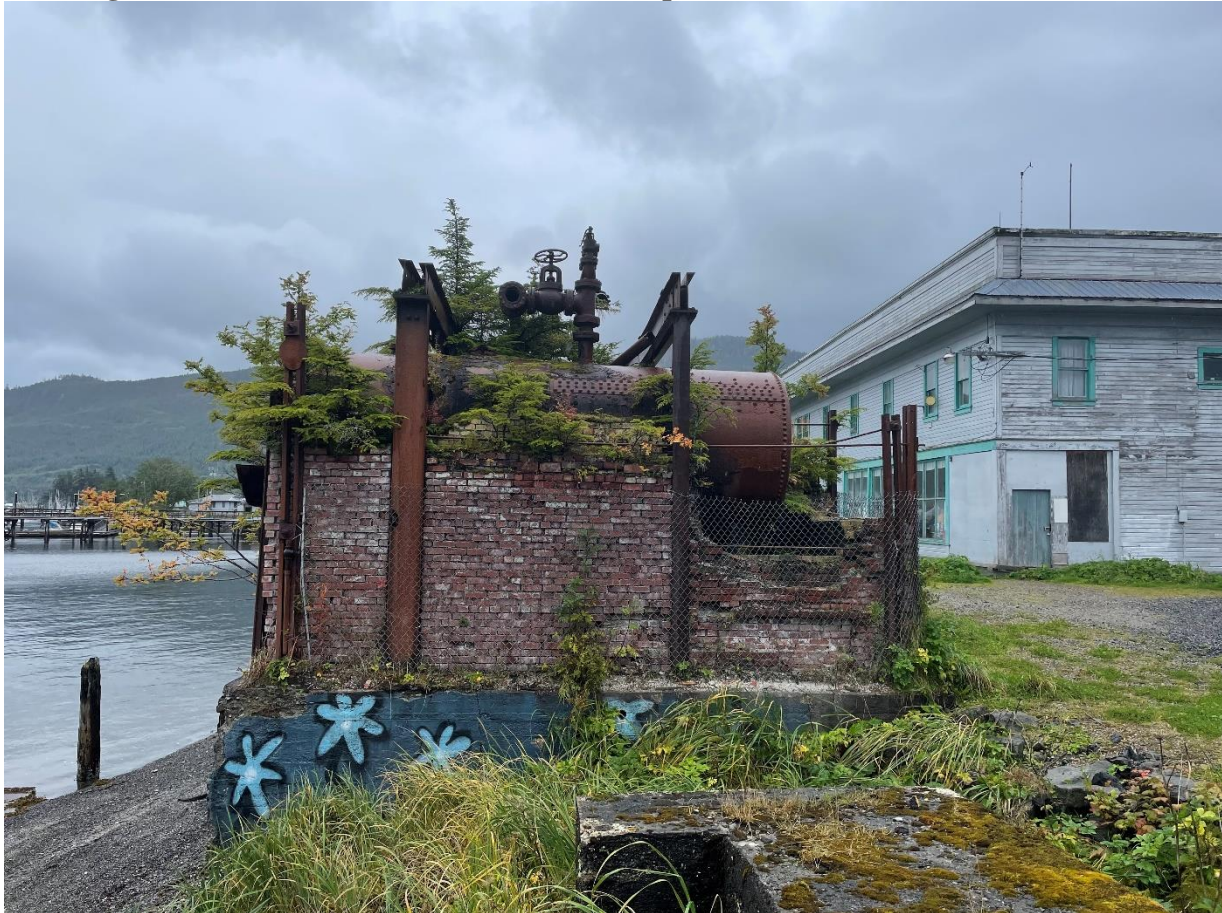
West side of steam plant
