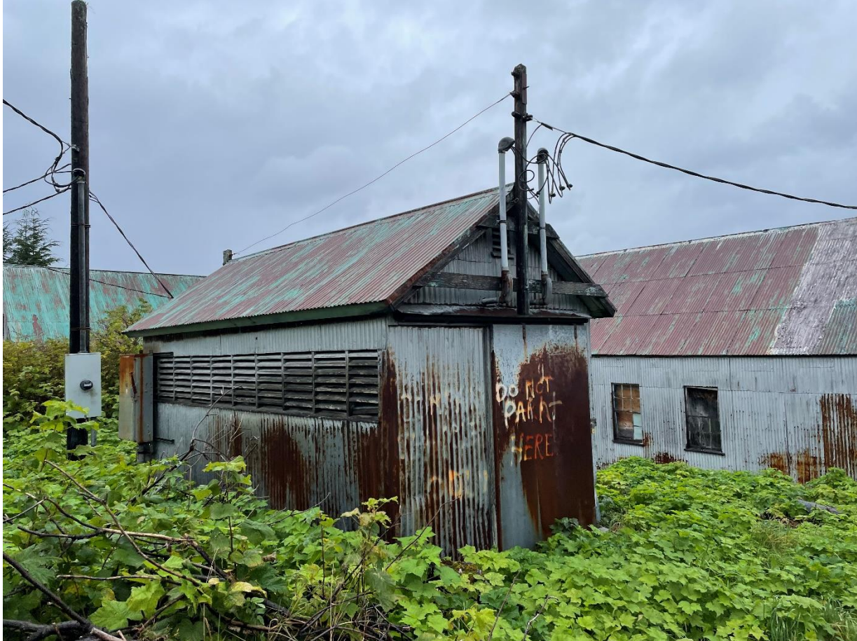
Southeast corner view
