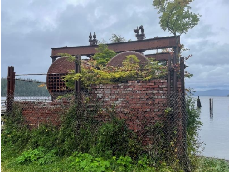
South side of steam plant
