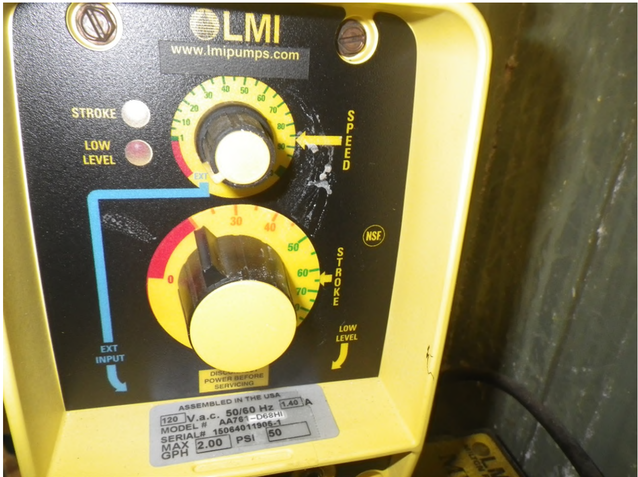
Figure 48 Chlorine pump
