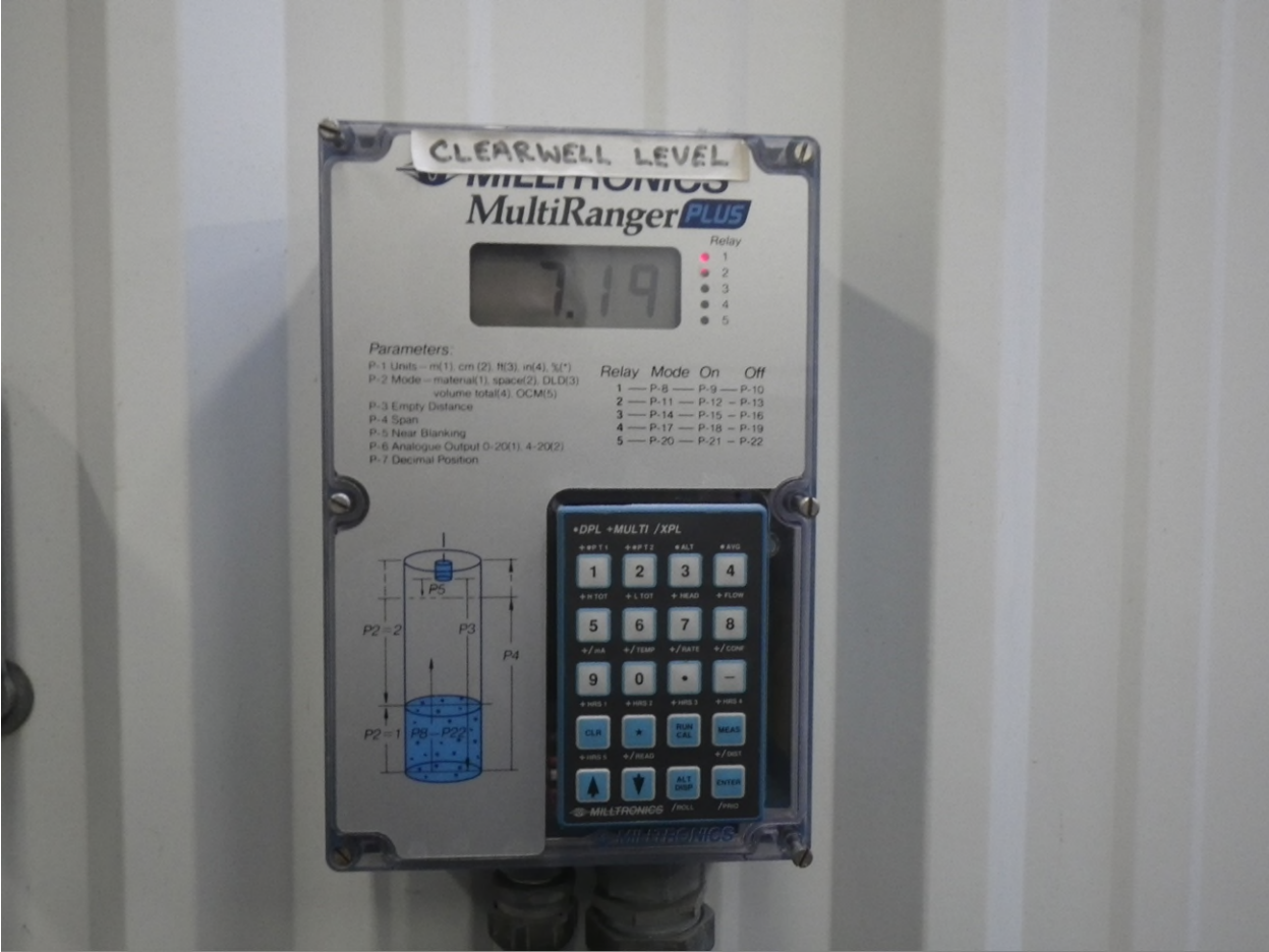
Figure 54 Clear well level
