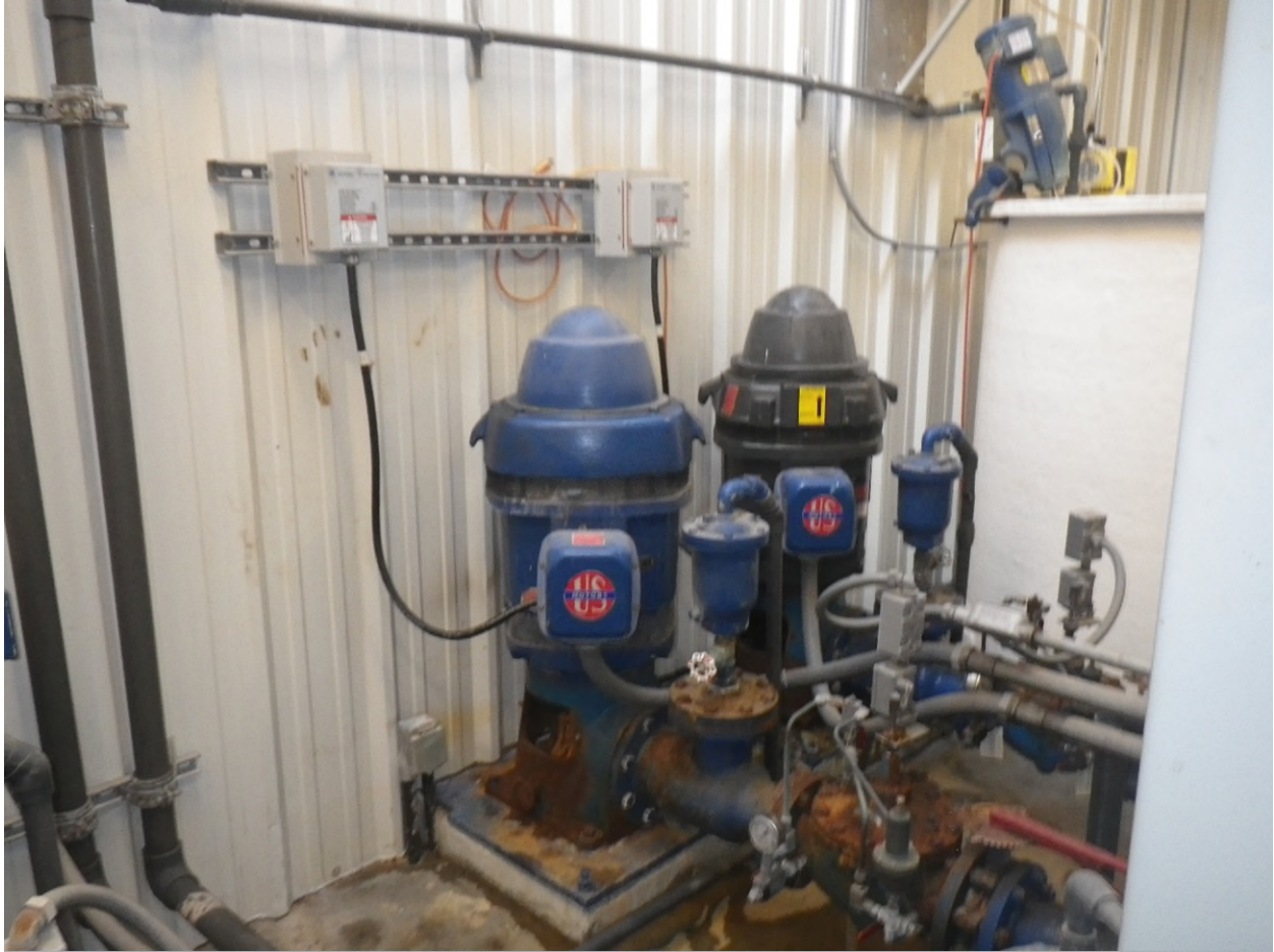
Figure 63 50 HP motors, both the same
