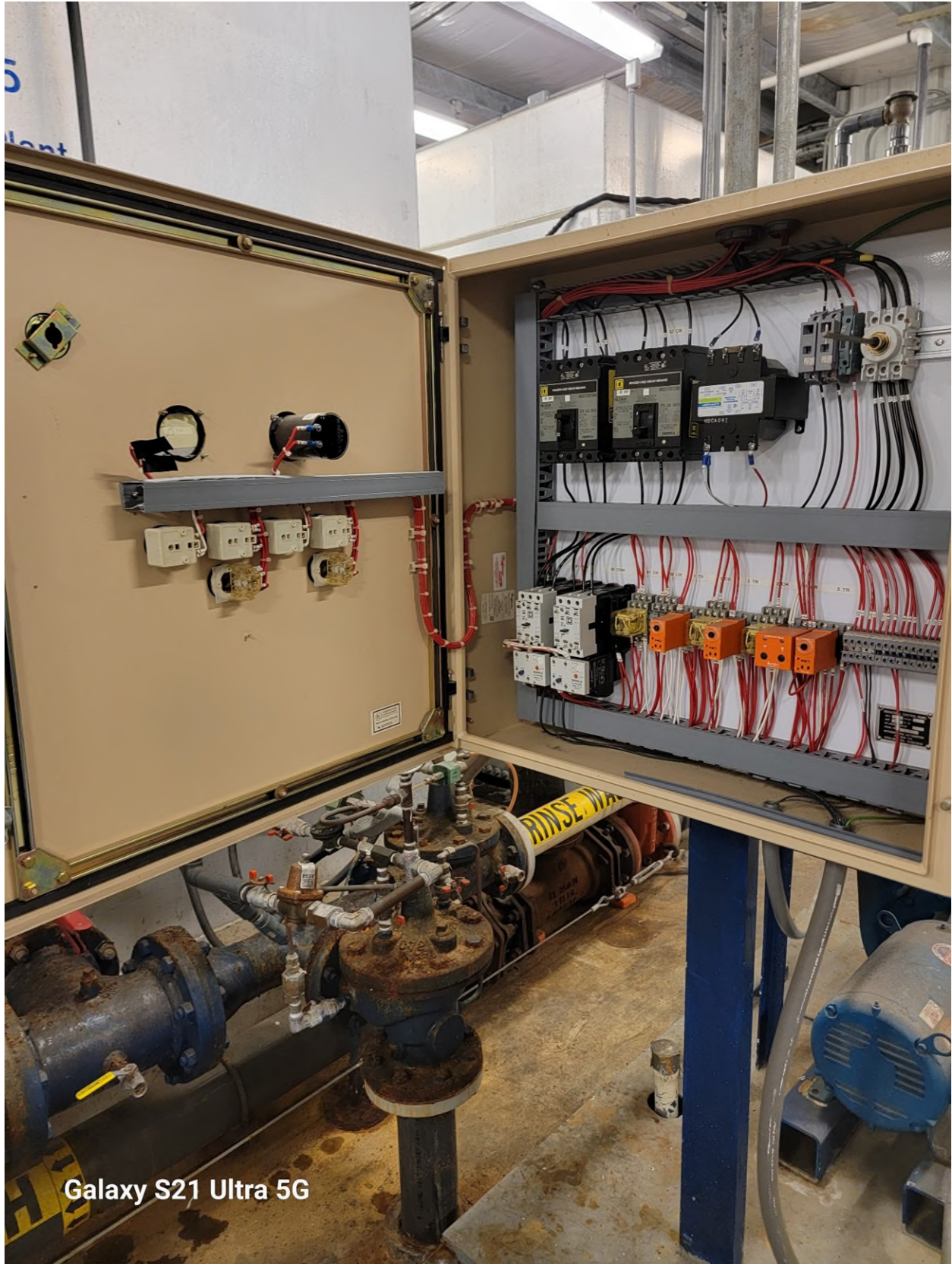
Figure 78 Backwash panel
