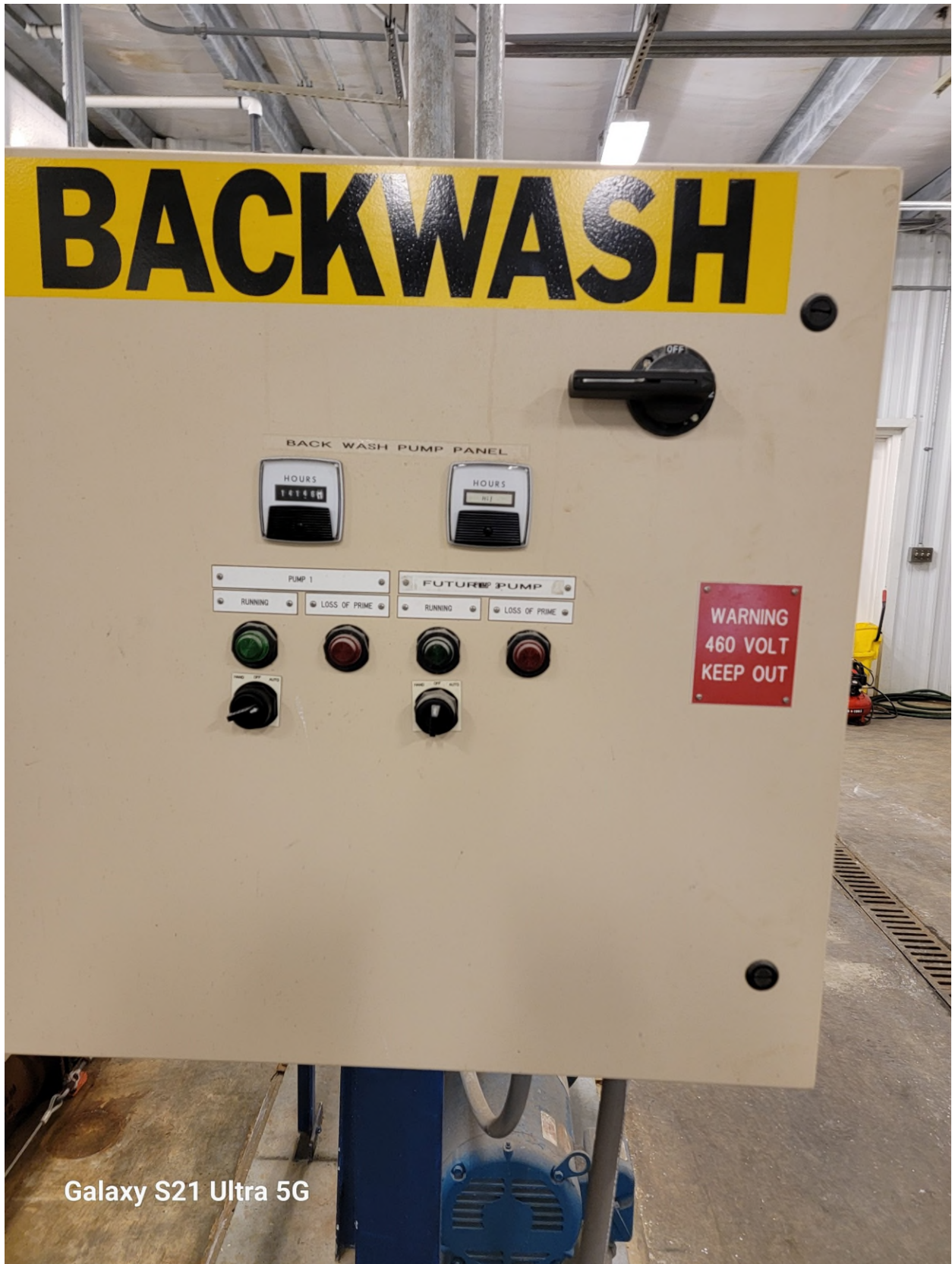
Figure 77 Backwash pump panel
