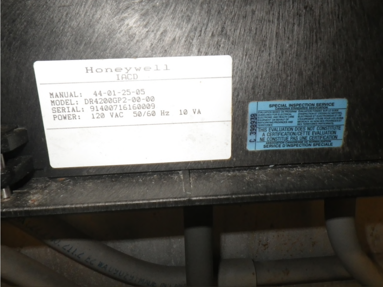
Figure 33 Chart recorder
