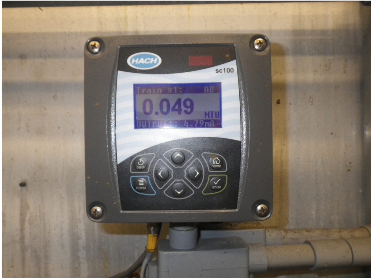
Figure 32 Turbidity controller, for 1720E turbidity meters
