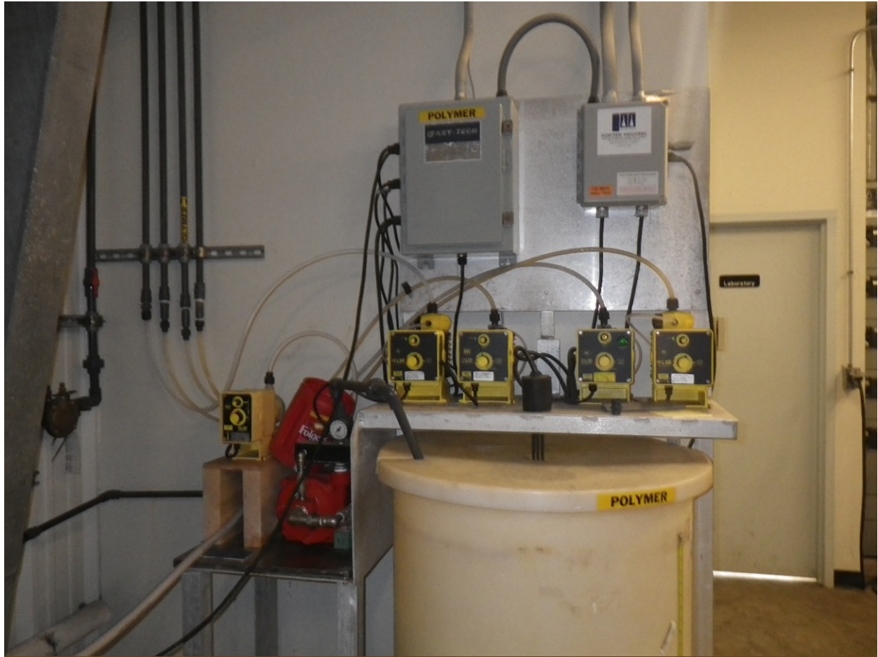
Figure 21 Polymer Station
