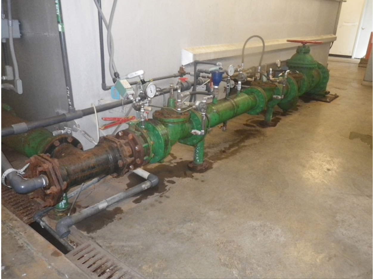
Figure 2 2 Prv's with PLC control flow
